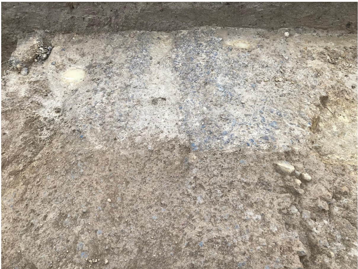
Fig (17) East facing Northern surface area of the road (A) showing cart wheel impressions into the metalized surface.
