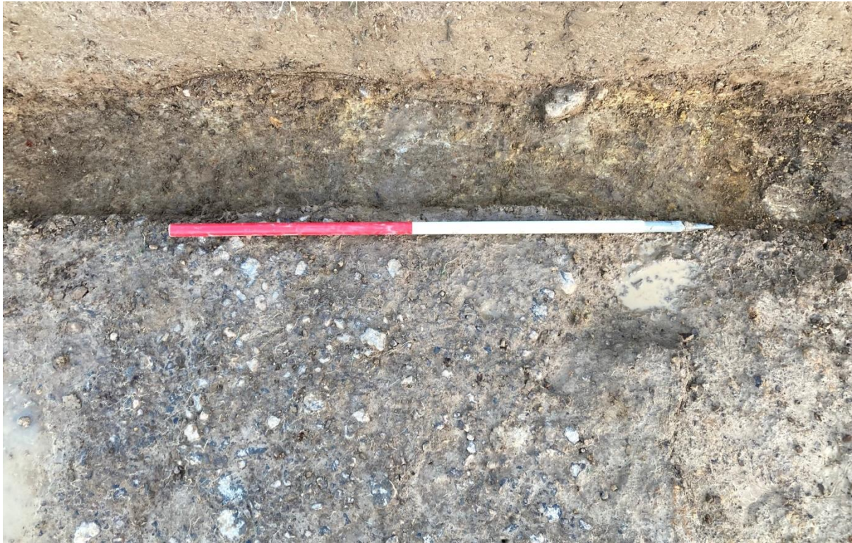
Fig (22) North facing section of the road surface (A) revealing the depth of the metal slag surface onto the natural sandstone and clay base.
