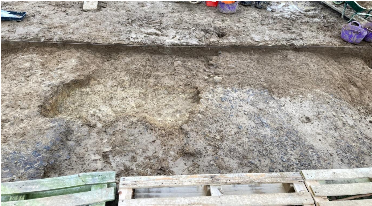
Fig (20) Historically removed central section of the road surface.
