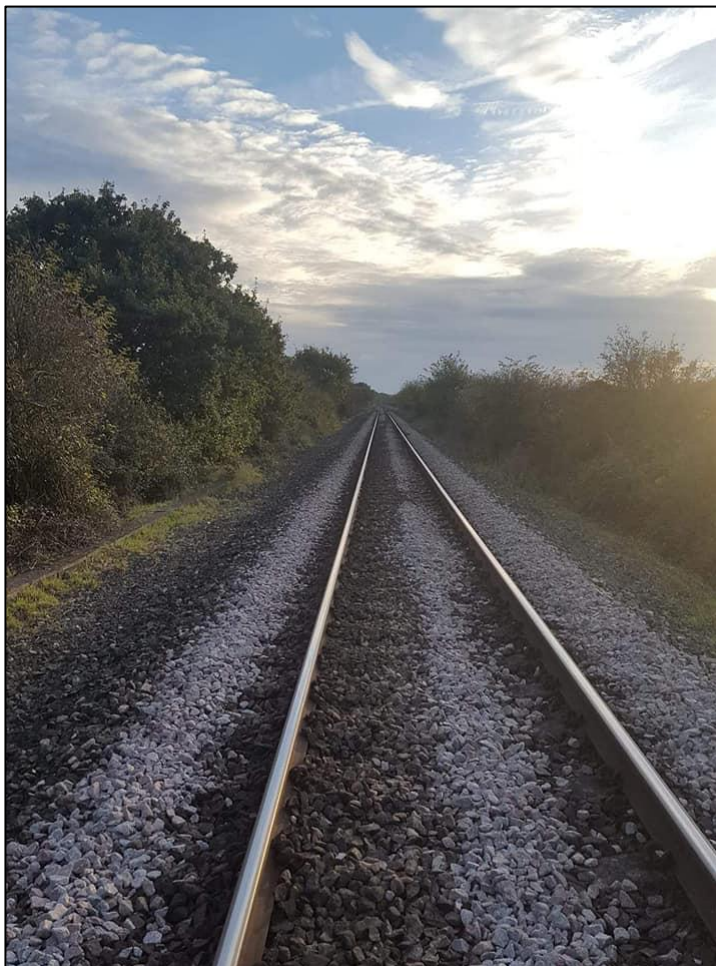
Rye railway view to Winchelsea Richard Hutley
