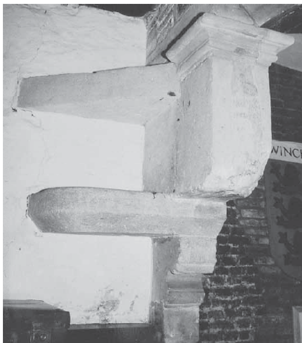
Fig. 11.25 The Court Hall, Quarter 8. South side of the fireplace showing the moulded corbels supporting the remains of the former ground-floor fireplace hood. Note the adjacent 'candle' shelves.
