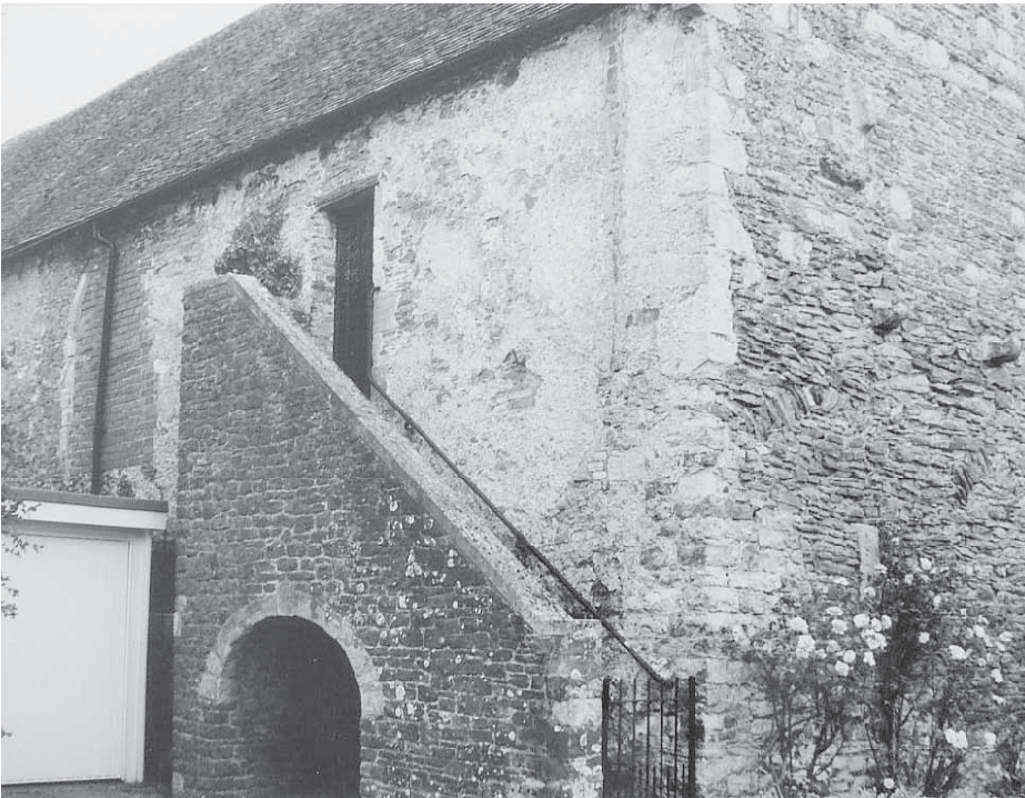
Fig. 6.2 (Left) The Court Hall. Exterior from the northwest showing the former internal northern wall with a blocked medieval first-floor doorway visible on the left and an intruded 16th-century first-floor doorway leading to rebuilt steps in the centre. Note how the quoins at the corner of the building terminate part way down the wall.
