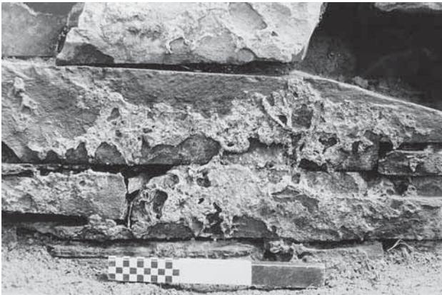
Fig. 5.11 Remains of lime render adhering to the face of the clay-bedded wall.
