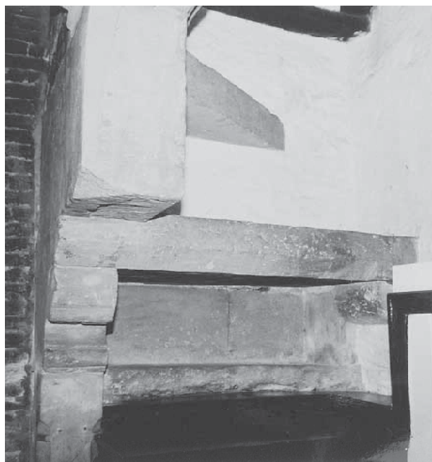
Fig. 11.26 The Court Hall, Quarter 8. North side of the fireplace showing the moulded corbels supporting the remains of the former ground-floor fireplace hood. Note the adjacent 'candle' shelves.
