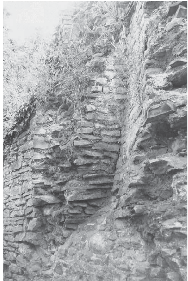
Fig. 11.33 Standing Gable, Quarter 2, North Street. Remains of the ground-floor fireplace showing the remains of the side jamb.
