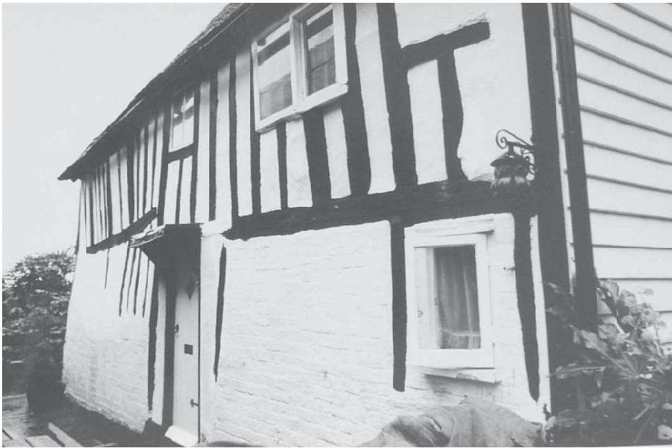
Fig. 11.10 (Left) Crowsnest, The Strand. Close-studding within the front elevation.
