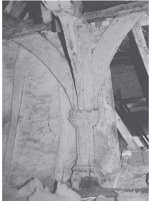
Fig. 11.18 Wren Cottage, Quarter 13. Formerly free-standing crownpost to the first-floor chamber.
