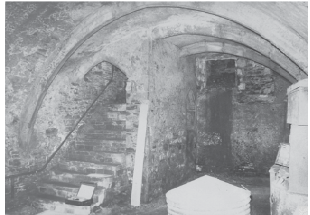
Below: Fig. 9.29 Cellar 4. A typical stair enclosure incorporated within the corner of the cellar. Note the cupboard recess in the right-hand side wall of the enclosure and the high-level window in the street facade (end wall) of the cellar.
