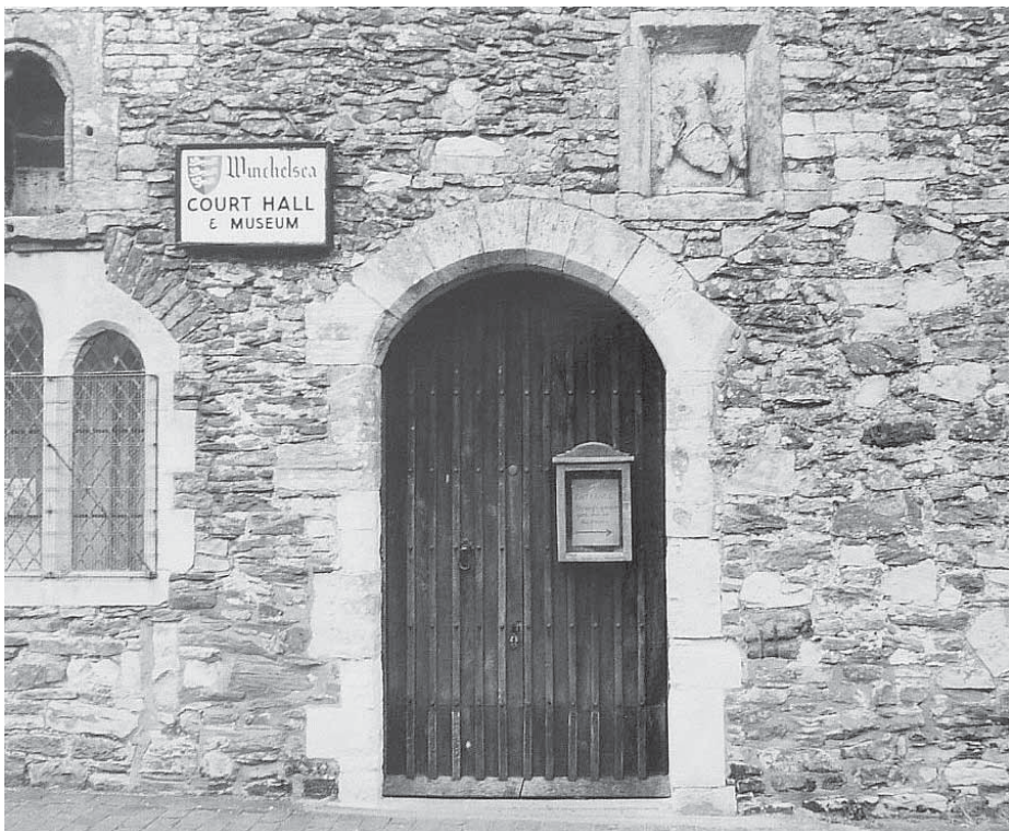
Fig. 6.3 (Left) The Court Hall. Intruded (probably 16th-century) external doorway in the south wall. Note the blocked window immediately to the right (evidence for it is one surviving voussoir and jamb stones shared with the doorway, and a scar in the masonry immediately above the removed voussoirs). Above the shared jamb of the doorway and window is a recessed plaque bearing a coat of arms.
