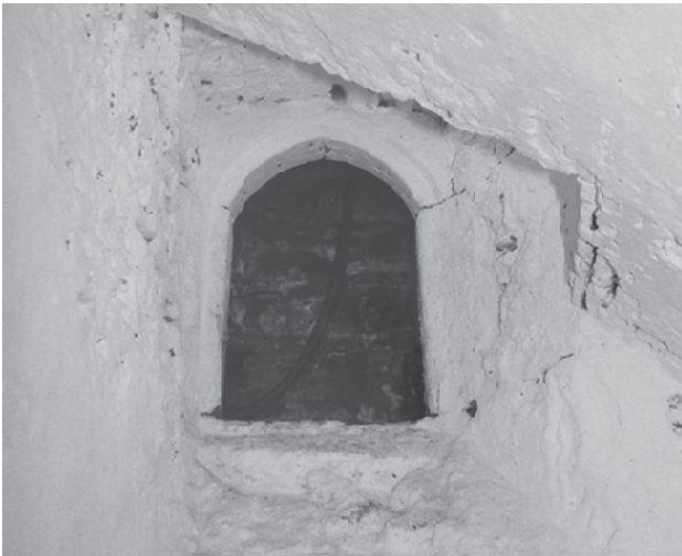
Fig. 9.19 Cellar 12. Detail of the window beside the entrance doorway.
