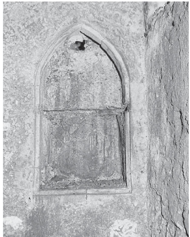
Fig. 9.38 Cellar 4. A typical cupboard recess with two-centred head. Note the impression of a former timber shelf.
