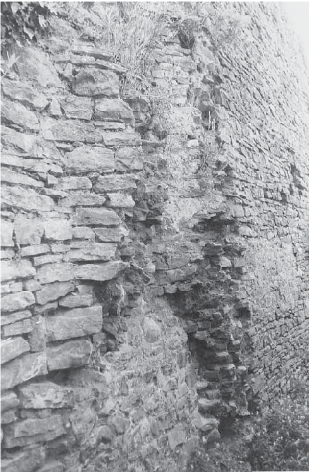
Fig. 11.32 Standing Gable, Quarter 2, North Street. Remains of the ground-floor fireplace showing the canted front wall.
