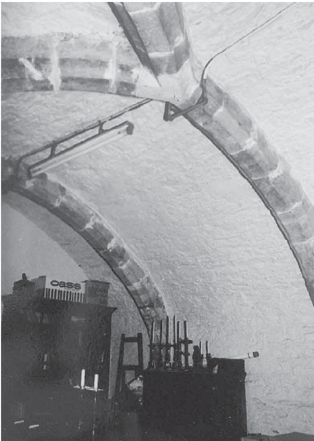
Fig. 7.9 St Thomas's Church. Crypt beneath the altar looking west and showing tripartite vaulting.
