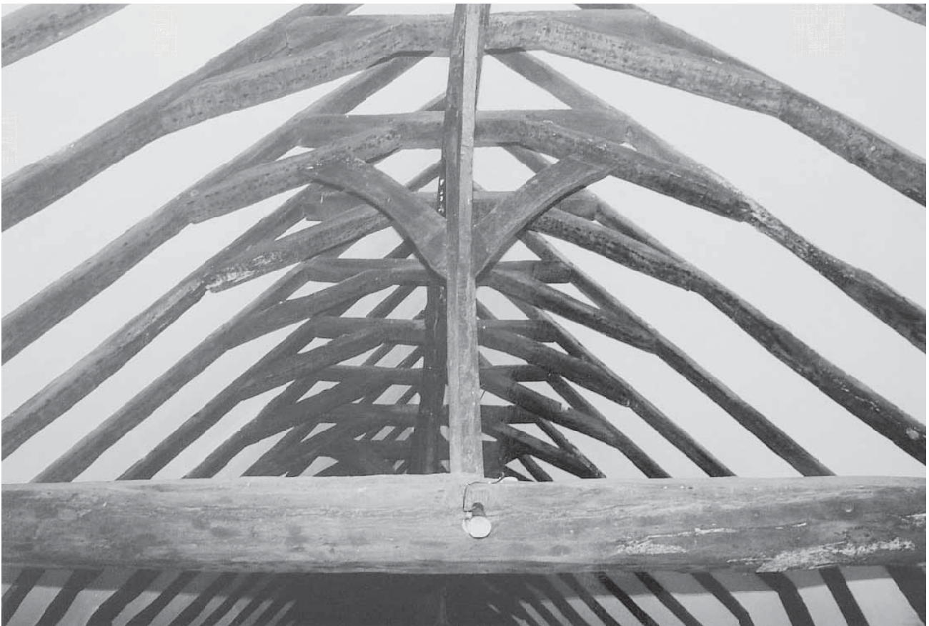
Fig. 6.1 The Court Hall. 15th-century crownpost roof.
