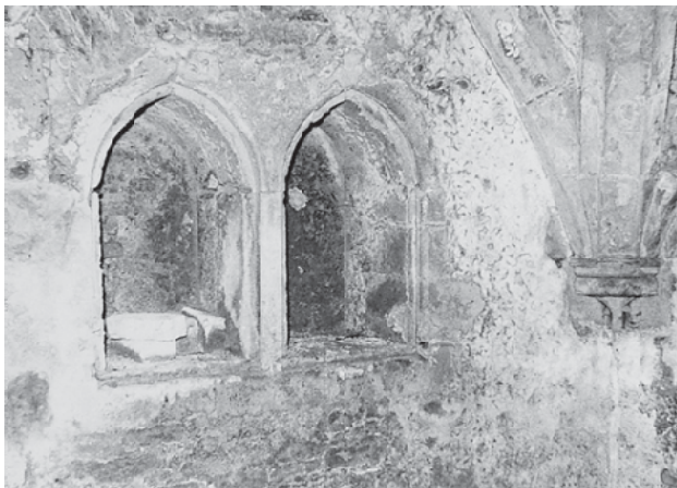
Fig. 9.37 Cellar 3. A pair of cupboard recesses with two-centred arched heads adjacent to the doorway in the west wall.
