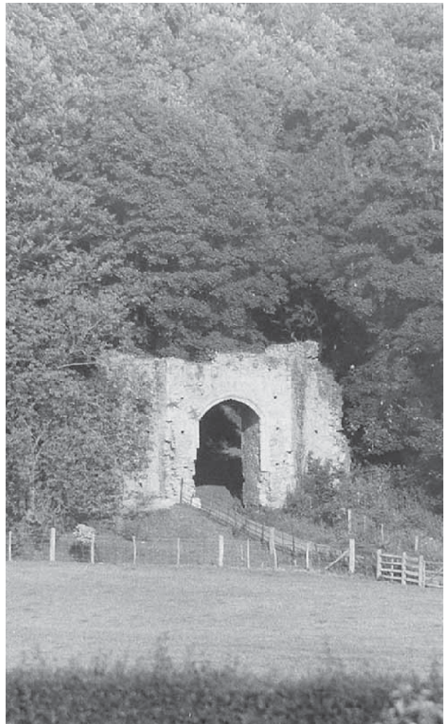
Fig. 5.23 New Gate viewed from the west showing its isolated rural location.
