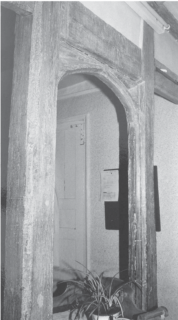
Fig. 11.13 Periteau House, Quarter 7. First-floor doorway showing a simple four-centred arched head.
