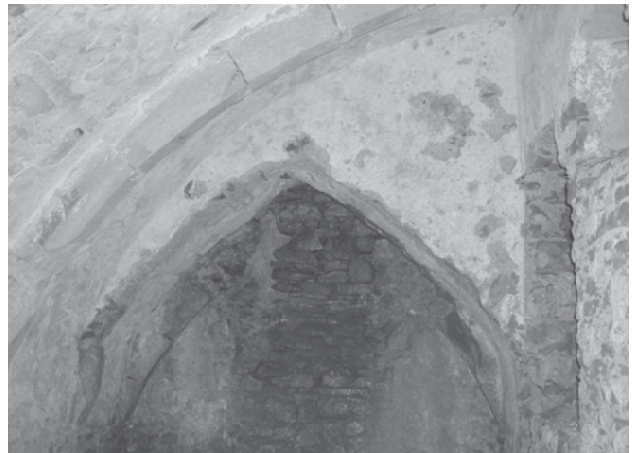
Fig. 9.22 Cellar 31. Arch supporting front wall of house.
