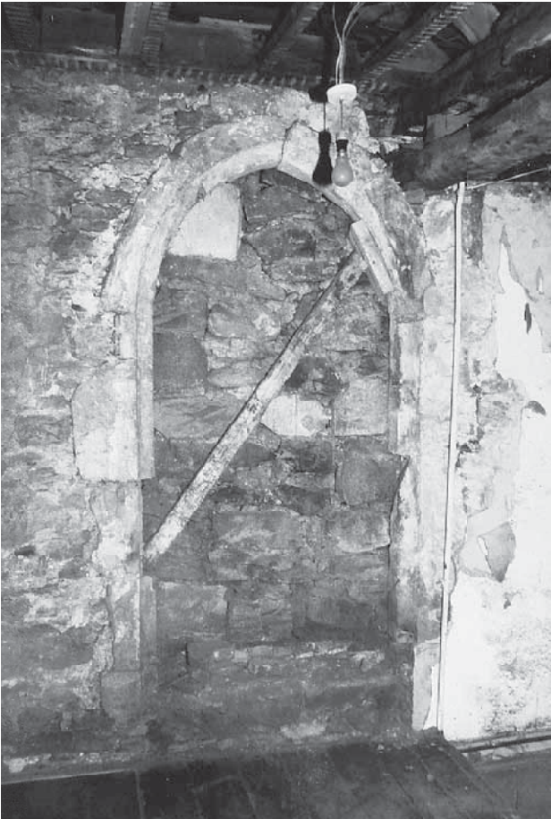
Fig. 11.3 Old Castle House, Quarter 8. First-floor doorway.
