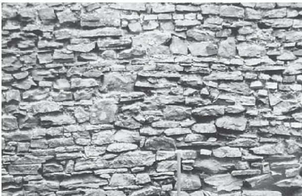
Fig. 11.1 Typical Tilgate stone wall at Blackfriars Barn.
