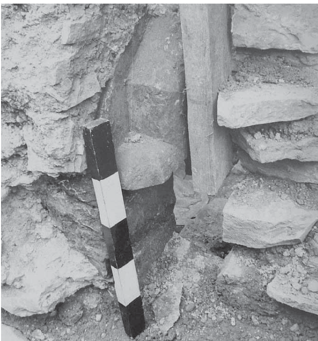
Fig. 9.26 Cellar 30. Return stop to the hood mould on the cellar window adjacent to the main entrance steps.
