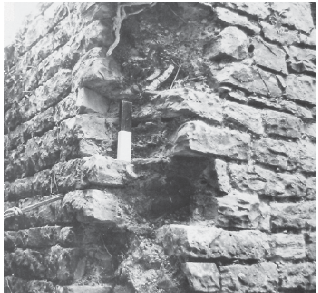
Fig. 11.2 Roughly squared facing blocks at the Standing Gable, Quarter 2.
