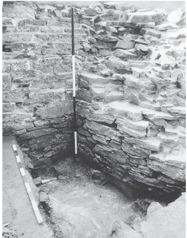
Fig. 5.12 Bonded junction between the turret 'C' (right) and the town wall (left).
